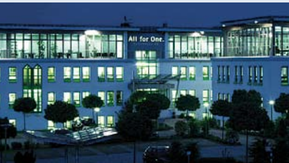
All for One Headquarters, Germany
